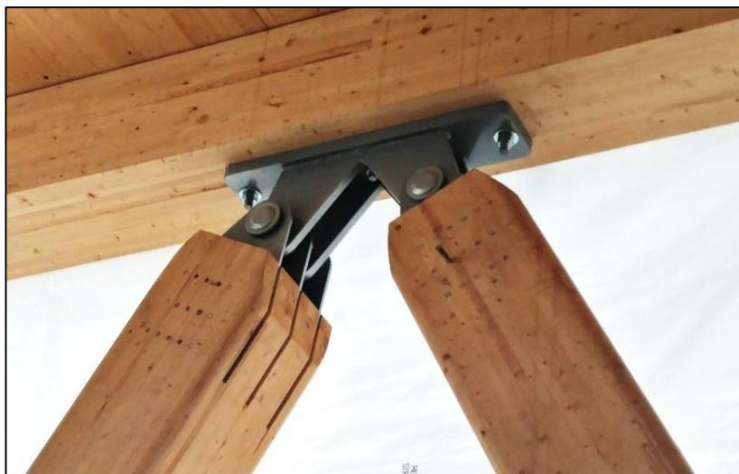
Figure 2-1: Example of bolted connection with multiple layers of steel
